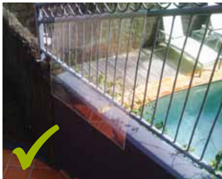
A flat polycarbonate sheet can be used to shield a climbable object.
