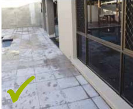
These windows have fixed security screens.
