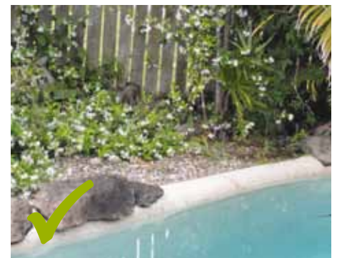
This garden bed does not reduce the fence height.
